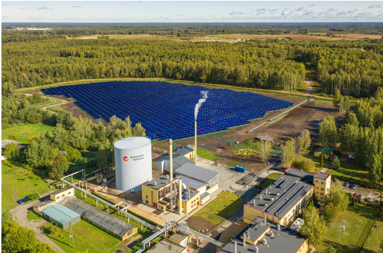
Latvia: 15 MW SDH plant (21,672 m 2 ) inaugurated at 12 September 2019 (photo: Salaspils Siltums)
