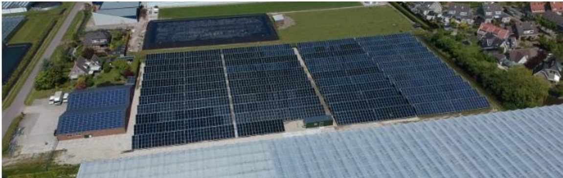
October 2019, 9,300 m 2 (6.5 MW th ) flat plate collectors supply heat to freesias greenhouse farm in Northern Netherlands (photo: G2Energy )
