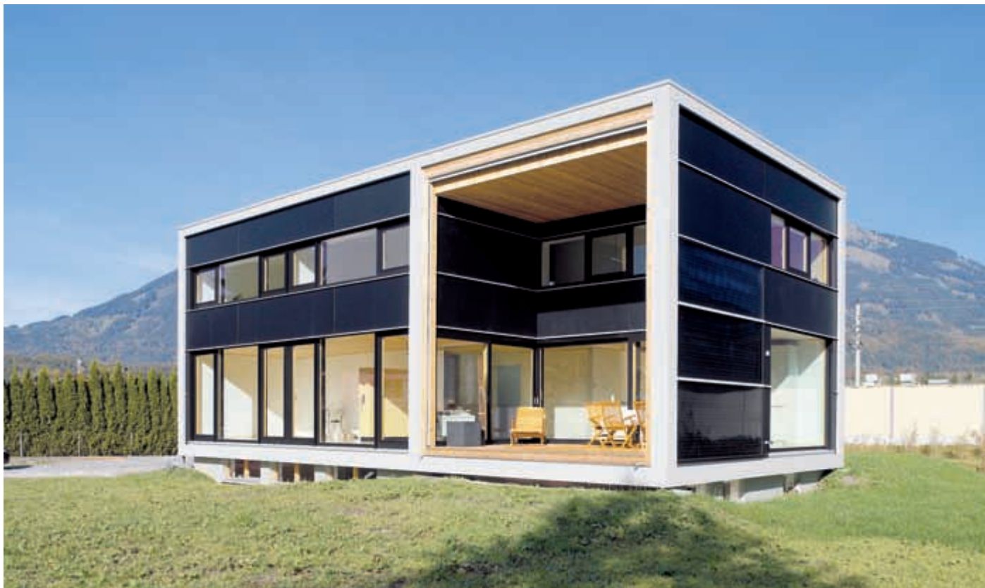
A 12 m 2 hot water system is hidden in the façade of this modern residential building. The large-scale wood framed collectors come from Doma Solartechnik in Vorarlberg, Austria, which was acquired by the Swiss company Ernst Schweizer in March 2013.
