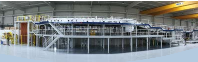
Production line in Bernburg, specially designed for roll-coating PVD process based on sputtering and electronic beam technology.
